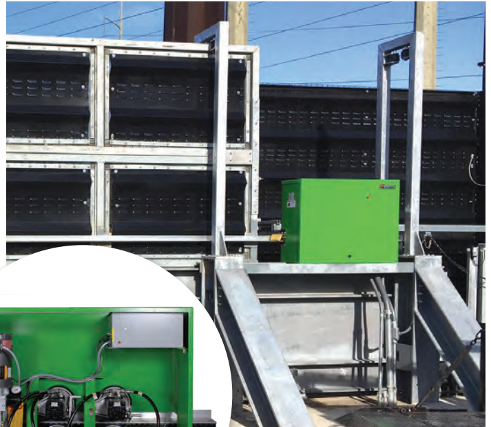
SlideDriver 200 operates crash gate at power substation
